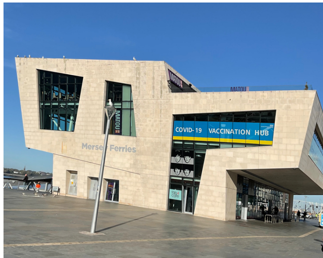
Pier head ticket office front view
