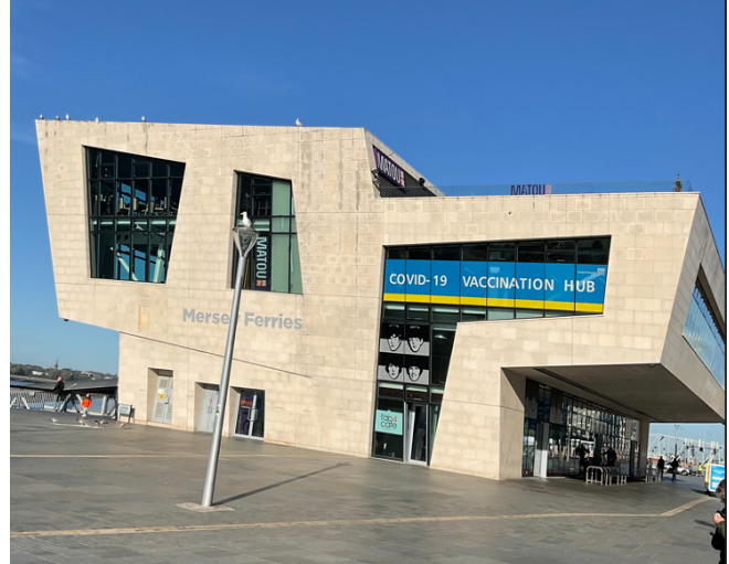
Pier head ticket office front view
