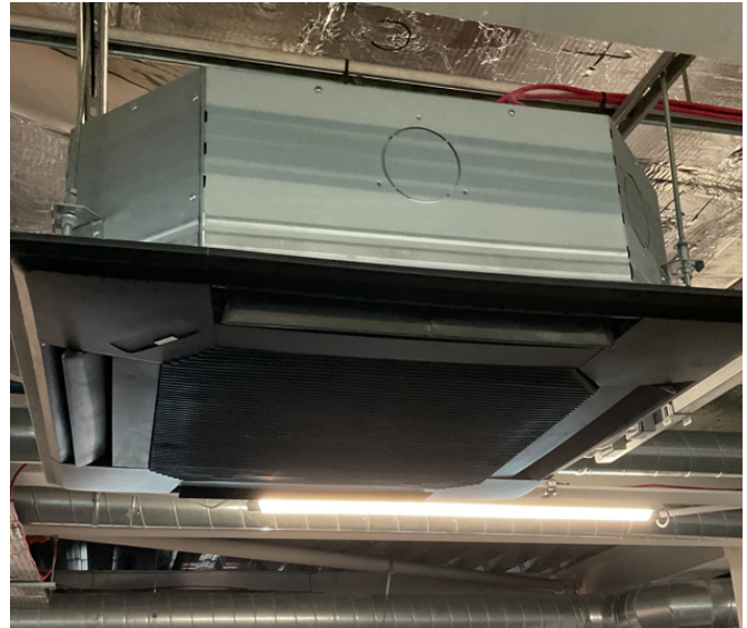
Air conditioning unit - Ceiling mounted cassette
