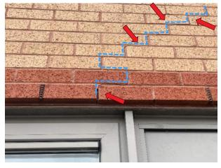
Figure 5, Hairline crack following a stepped pattern in the mortar.
