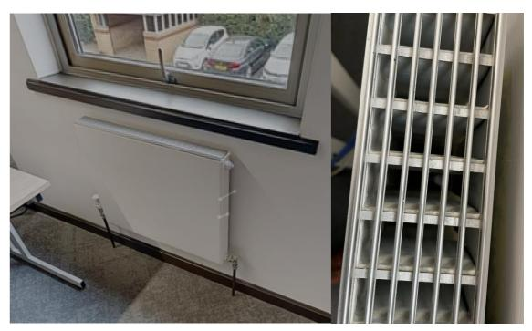
Figure 9 Typical office double panel radiator with fins.
