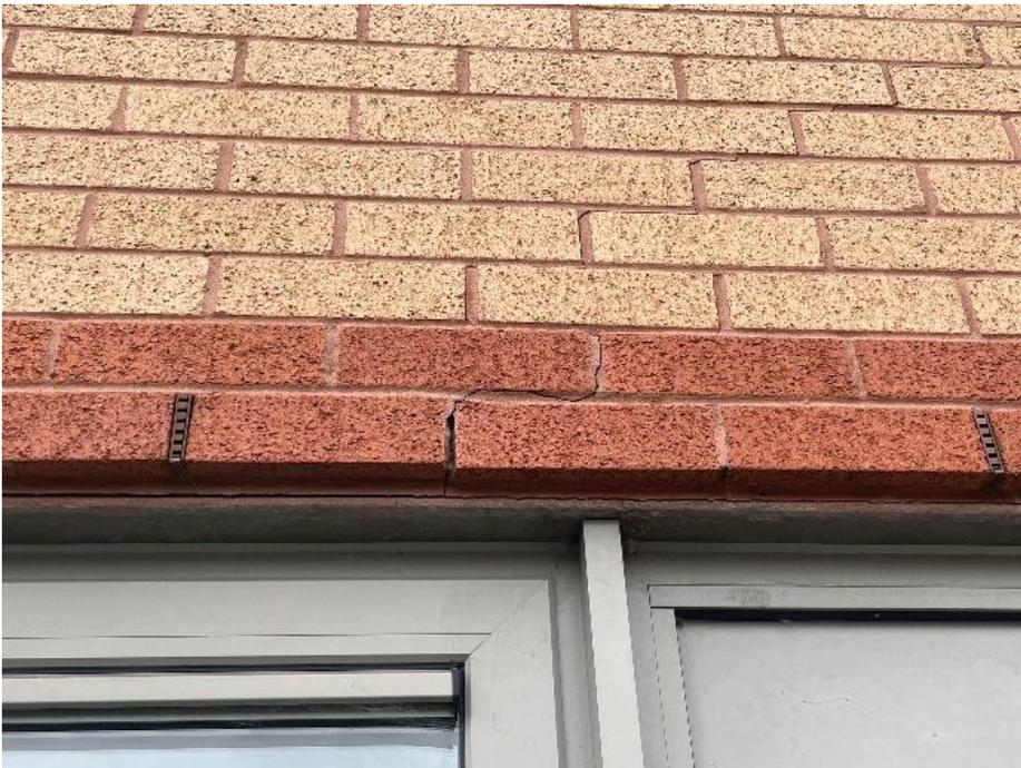
**Figure 3, Hairline crack observed in mortar above opening.**
