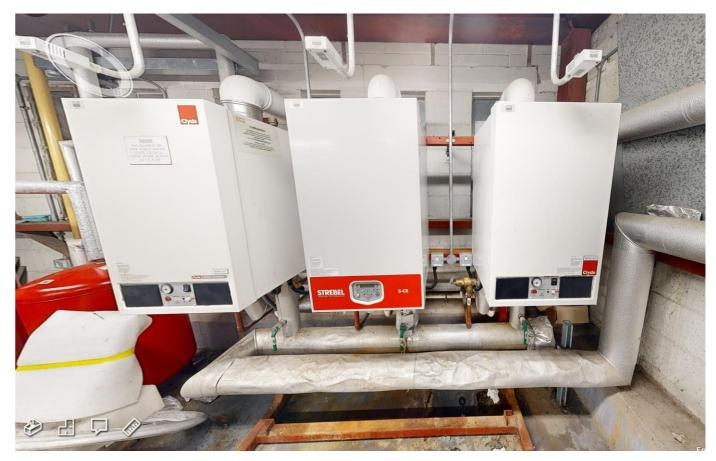
Figure 8 Existing gas fired boilers in roof heating plantroom
