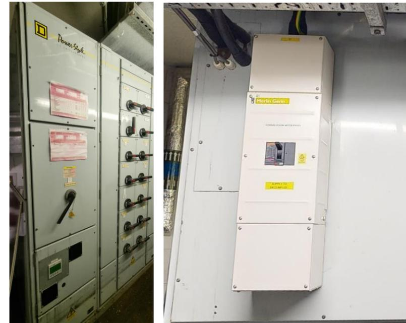
Figure 15 LV main switch panel (left) and image of additional outgoing feed (right)
