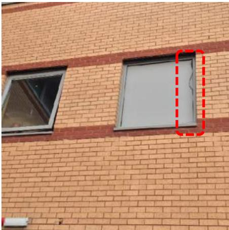
**Figure 28, gasket peeling from level 1 window**
