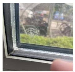
Figure 30, Glass marking on the internal face of windows
