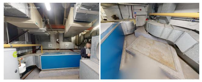
Figure 11 Existing AHU (left) and high level extract fans in the roof ventilation plantroom and the floor soft spot (right)
