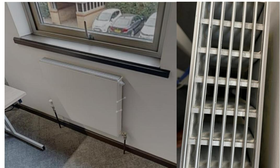
**Figure 9 Typical office double panel radiator with fins.**
