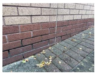
Figure 9, Evidence of consistent DPC location elsewhere.
