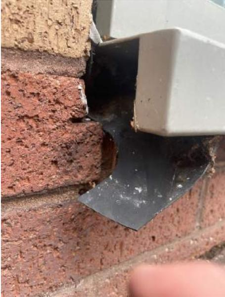
**Figure 20, Membrane below curtain wall sill**
