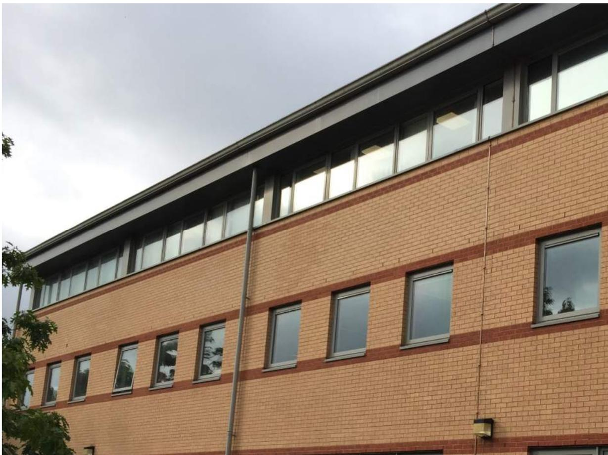
Figure 24, External view of punch windows and ribbon windows on level 1 and 2.
