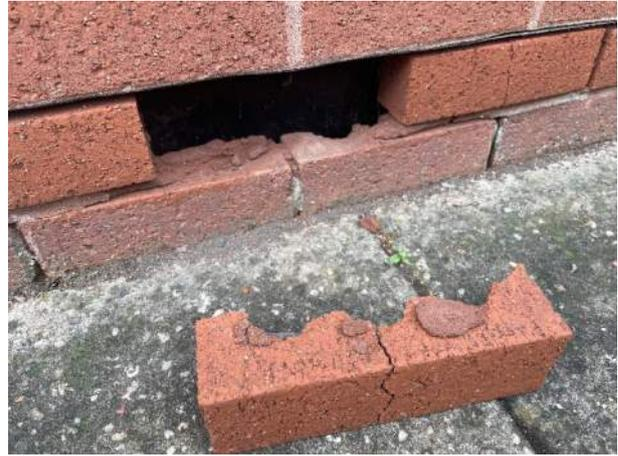
**Figure 11, Damaged half-brick below DPC.**
