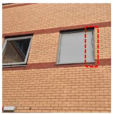
**Figure 28, gasket peeling from level 1 window** Gasket peeling is observed at multiple locations. Loose
