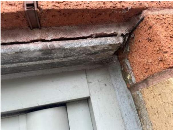
**Figure 18, Lintel corrosion at the head of opening.**
