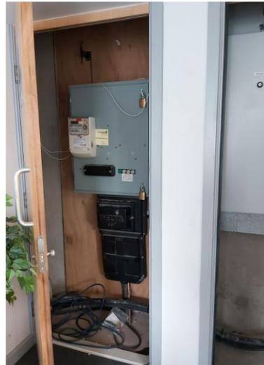
Figure 14 Electrical cut-out and metering equipment
