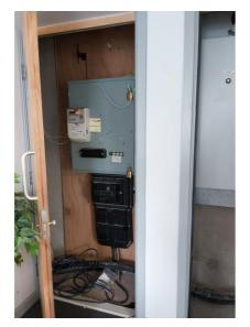
Figure 14 Electrical cut-out and metering equipment
