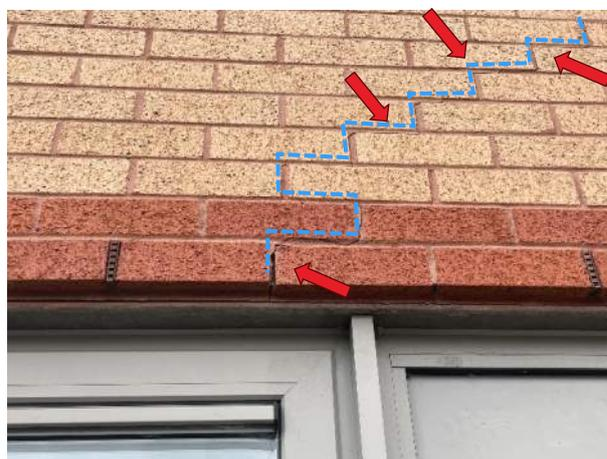
**Figure 5, Hairline crack following a stepped pattern in the mortar.**
