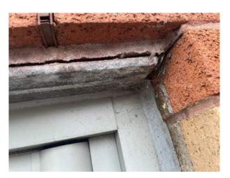
Figure 18, Lintel corrosion at the head of opening.
