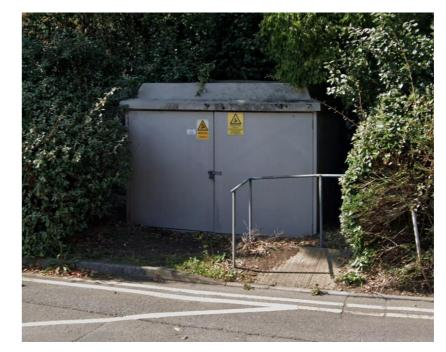
Figure 17 Existing Package Substation Enclosure
