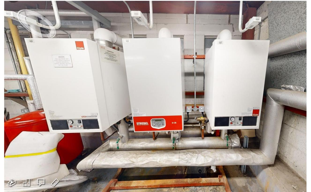
**Figure 8 Existing gas fired boilers in roof heating plantroom**
