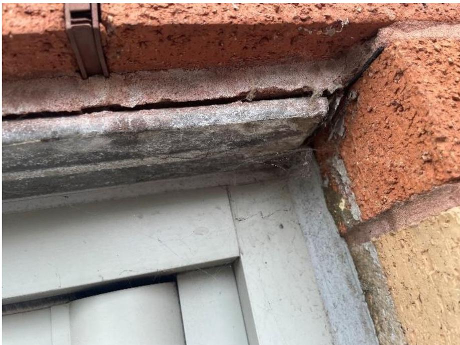
**Figure 2, lintel separation from brickwork above at the head of opening.**
