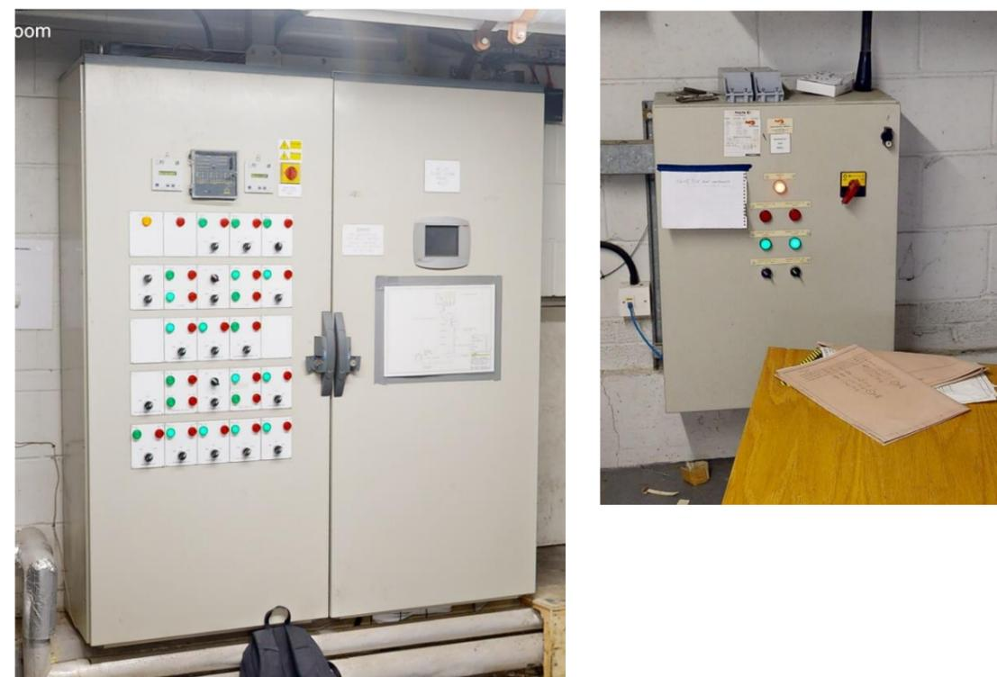
**Figure 13 Existing heating plantroom MCP (left) and basement plantroom MCP (right)**
