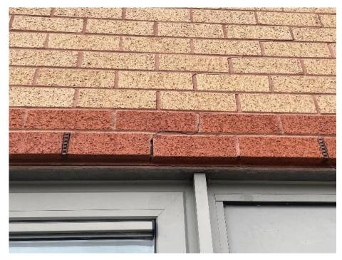
Figure 3, Hairline crack observed in mortar above opening.
