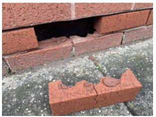
Figure 11, Damaged half-brick below DPC.
