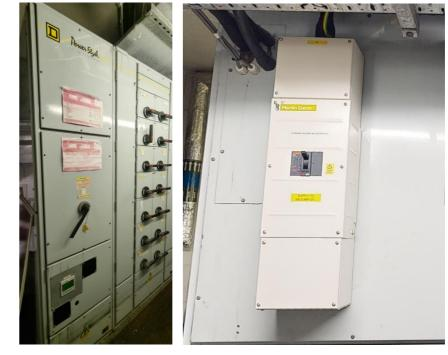
Figure 15 LV main swich panel (left) and image of additional outoing feed (right)
