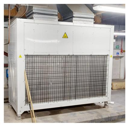
Figure 10 Existing ducted chiller in roof heating plantroom
