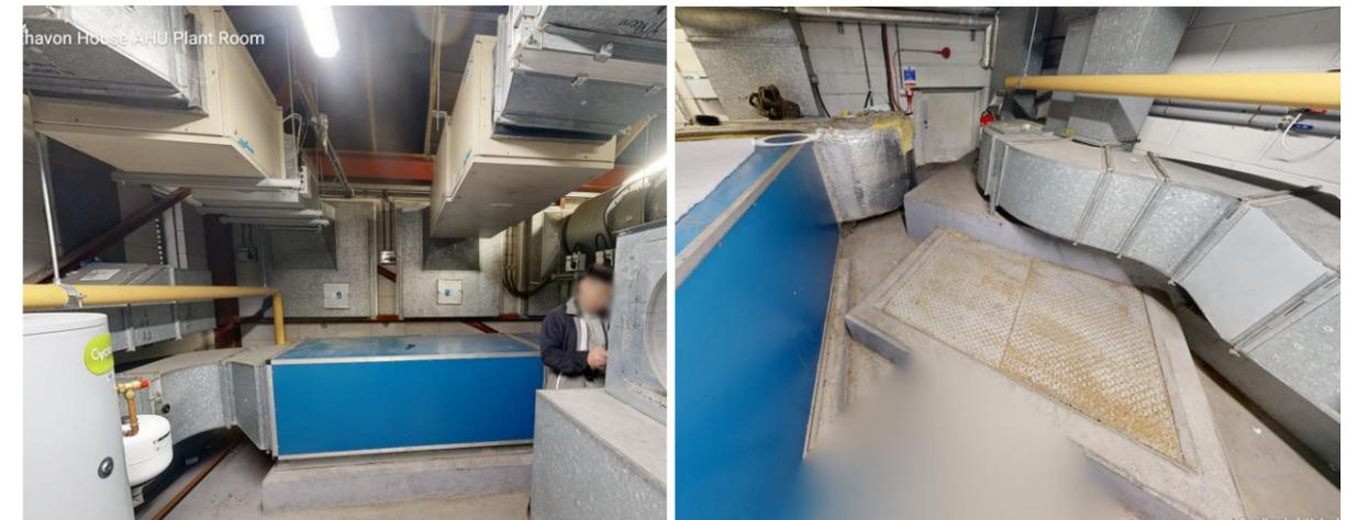
Figure 11 Existing AHU (left) and high level extract fans in the roof ventilation plantroom and the floor soft spot (right)
