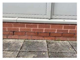
**Figure 10, Missing mortar below DPC.** Below the DPC, mortar is notably missing or loose.
