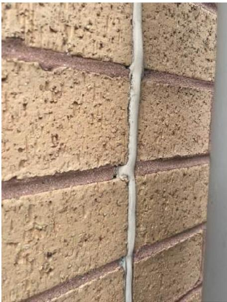
**Figure 12, Hardened silicone joint.**
