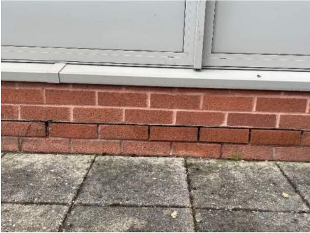
**Figure 10, Missing mortar below DPC.**
