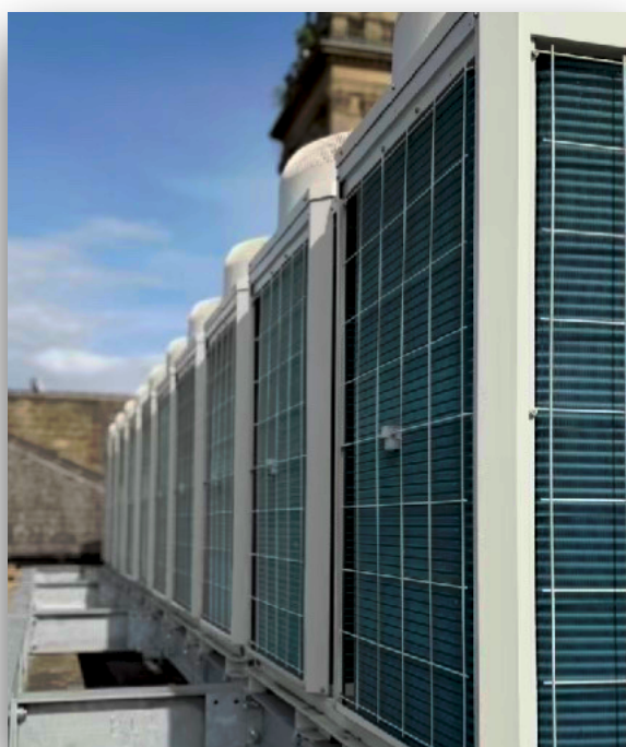
Air source heat pumps at Morley Town Hall installed with Public Sector Decarbonisation Scheme money.
