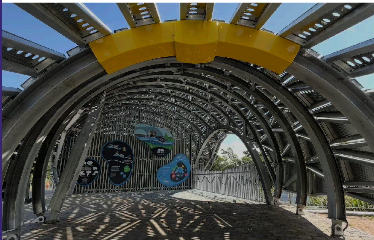
The 93kW twin-turbine 'Hydro Ness' hydroelectric generation system in Inverness
