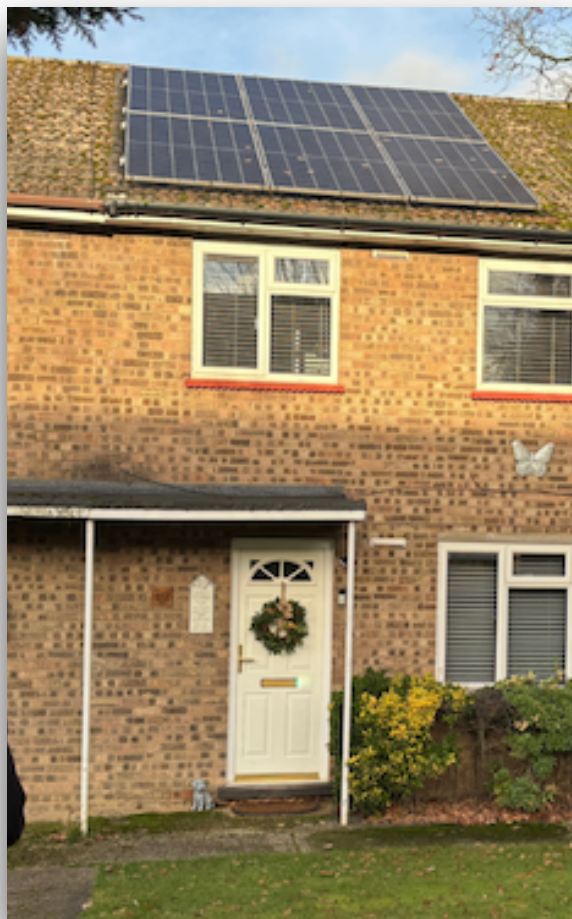
One of more than 100 homes in the borough of Colchester which have been upgraded with energy efficiency measures courtesy of Wave 2.1 of the Social Housing Decarbonisation Fund.
