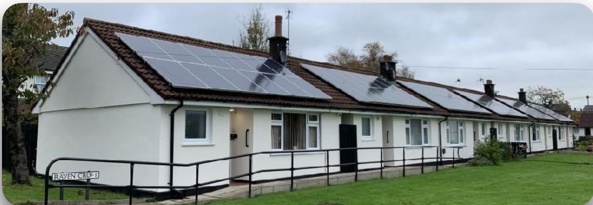
New solar panels installed on social housing at Raven Croft, Helmshore, Lancashire Picture credit: Together Housing Association.
