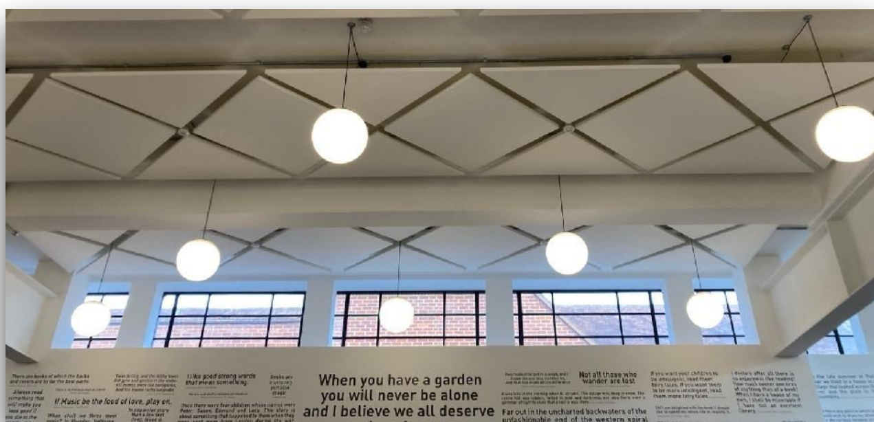
New LED lighting installed at Hillingdon Civic Centre. It was one of several Hillingdon Council projects which benefitted from £13.7 million of funding through Phase 3b of the Public Sector Decarbonisation Scheme.
