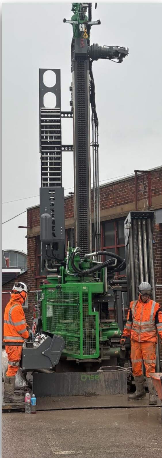
A borehole being drilled at Cranfield University which is harnessing a £7.8 million Public Sector Decarbonisation Scheme grant to replace its fossil-fuelled boilers with a ground source heat system.
