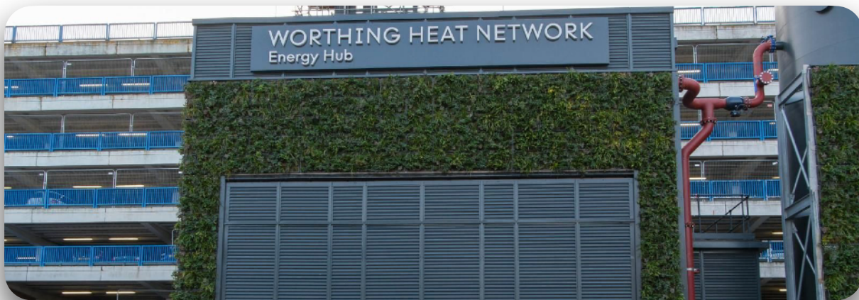
Worthing heat network central energy hub
