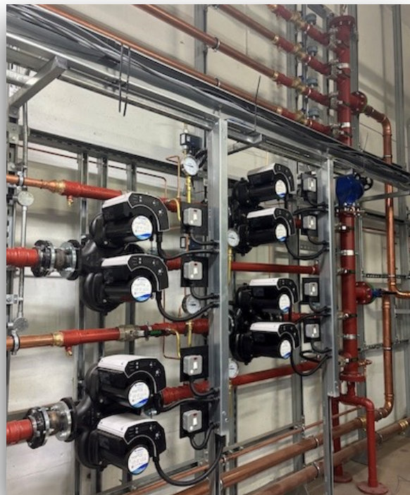
New heating controls installed at Lincoln College. The institution has benefitted from a total of £2.6 million from phases 3c and 4 of the Public Sector Decarbonisation Scheme.
